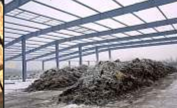
2 - open sided steel structure 9 000 m 2
