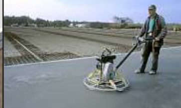
1 - reinforced concrete surface 8 100 m 2
