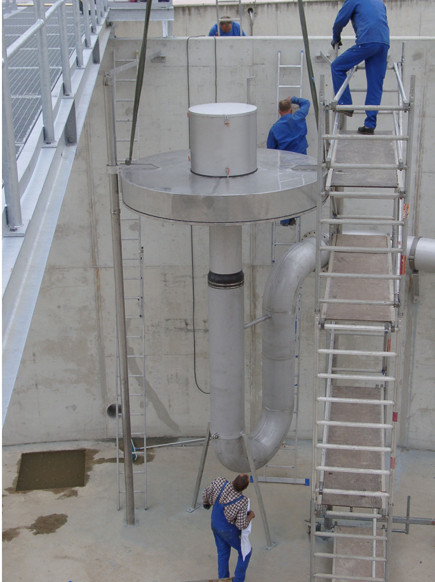
Figure 3: Lineardecanters (1,400 m 3 /h) during installation. The decanter heads are always floating in correspondence to the water level. The devices are closed during the SBR process and only opened to start the decantation step. The water removal is free of any suction, vortex or sludge ingress.
