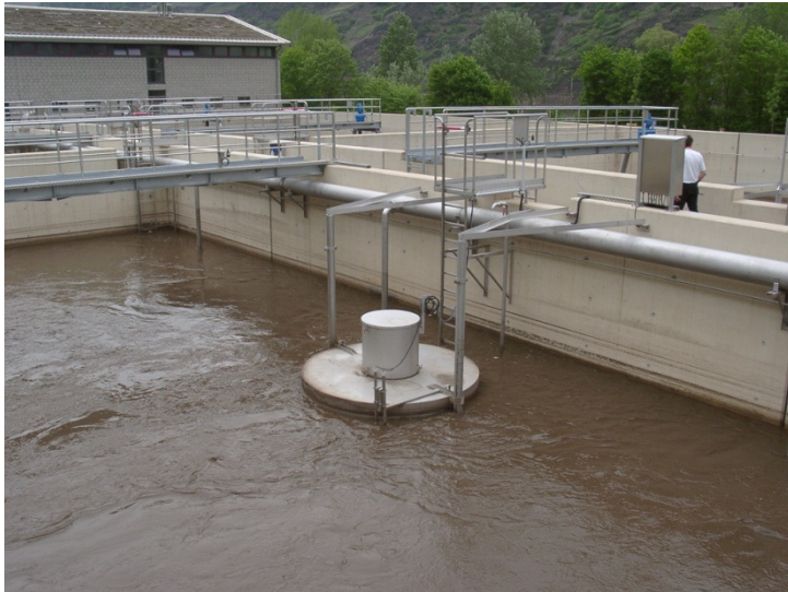
Figure 4: The Lineardecanter head during mixing
