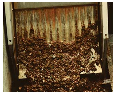
Typical photograph of the front face of a HYDRASIEVE® being used on slaughterhouse raw sewage. Notice clearly that the waste is concentrated at the bottom of the waves.
