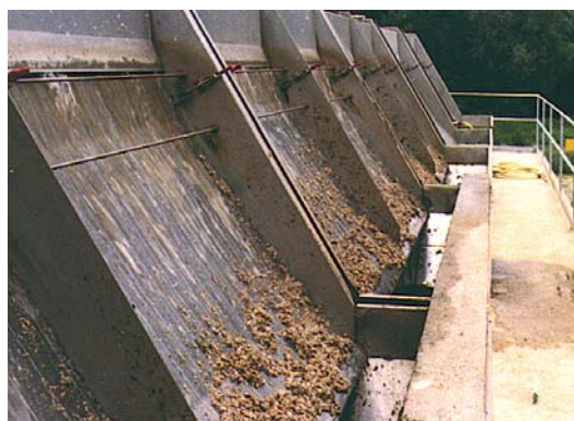
Raw municipal sewage. Stainless 554 frame - 3 x 96" and 2 x 72".
